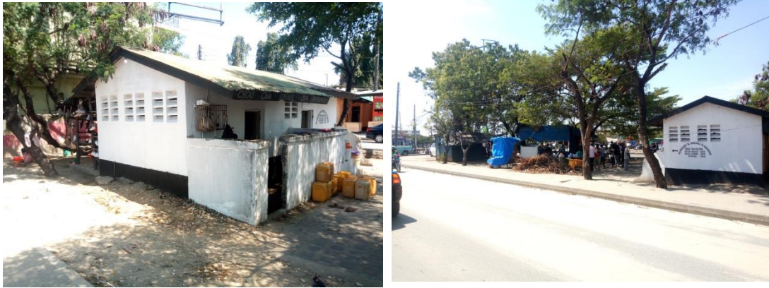
Figure 3: Artificial vegetation and structures at the project site
